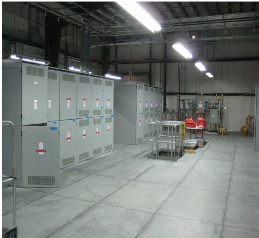
Fig. 3. Waste Treatment and Immobilization Plant Switchgear Building.
